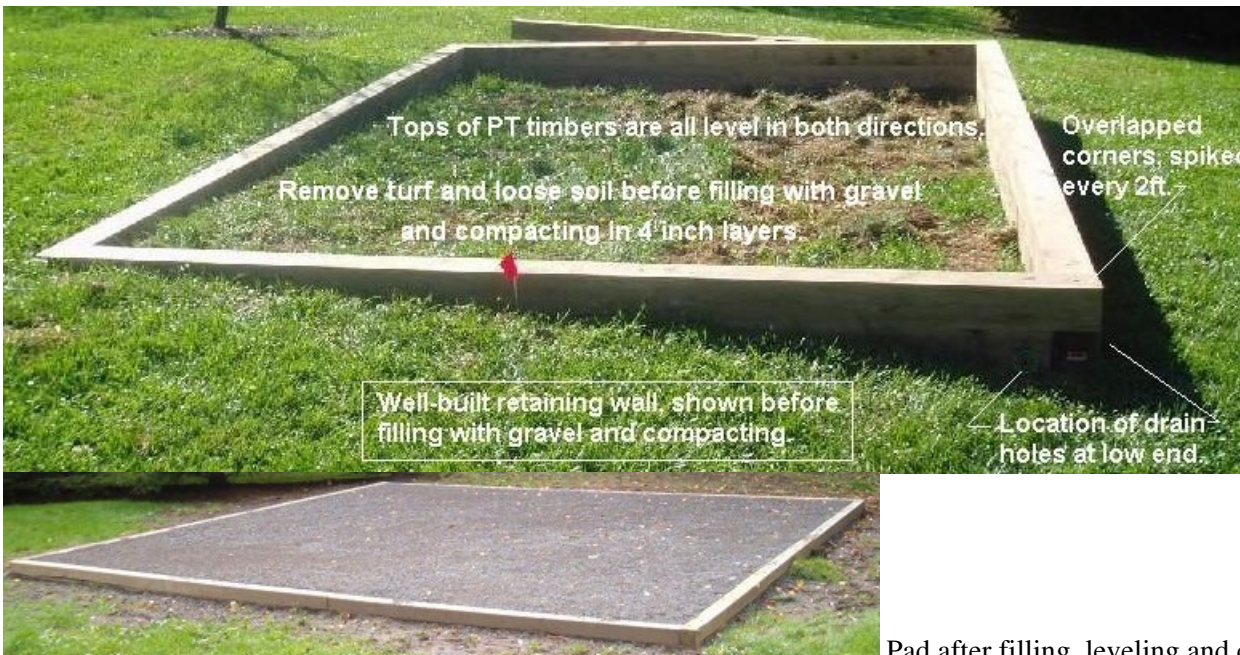
Pad after filling, leveling and compaction.
