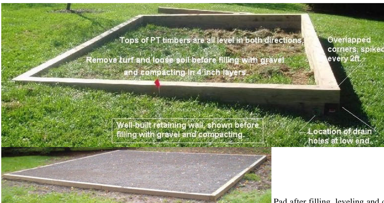
Pad after filling, leveling and compaction.
